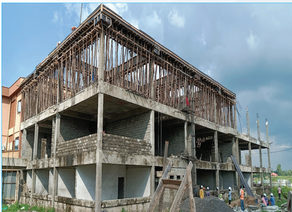
Figure 5: Health Science Laboratory Building at ring beam level (46% completion rate)
